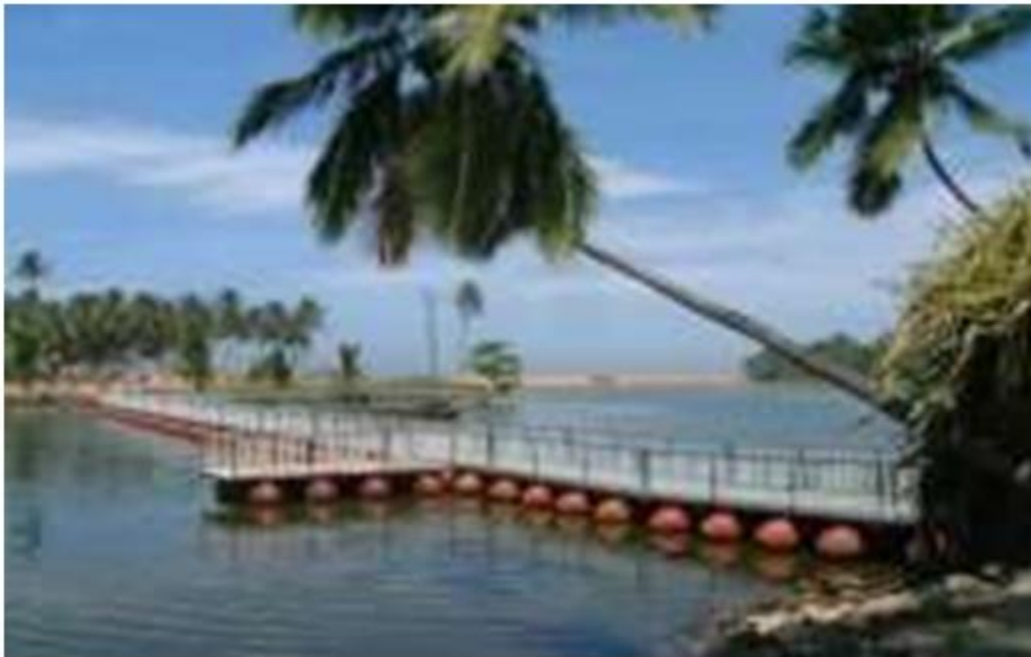
Figure 3: Floating Bridge in Veli
