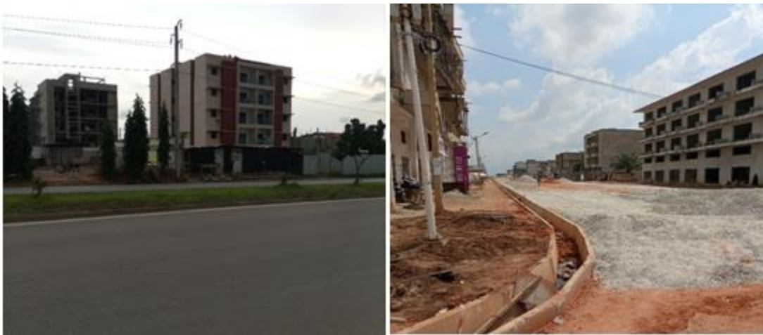
Figure 2. View of the buildings being finished near the UHC (Kobenon, 2020)
