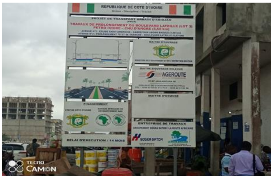
Figure 3. View of a plaque announcing the construction of service roads for the UHC (Kobenan, 2021)
