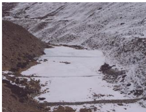
Figure 4: Simple Artificial Glacier Method (Source: LNP)
