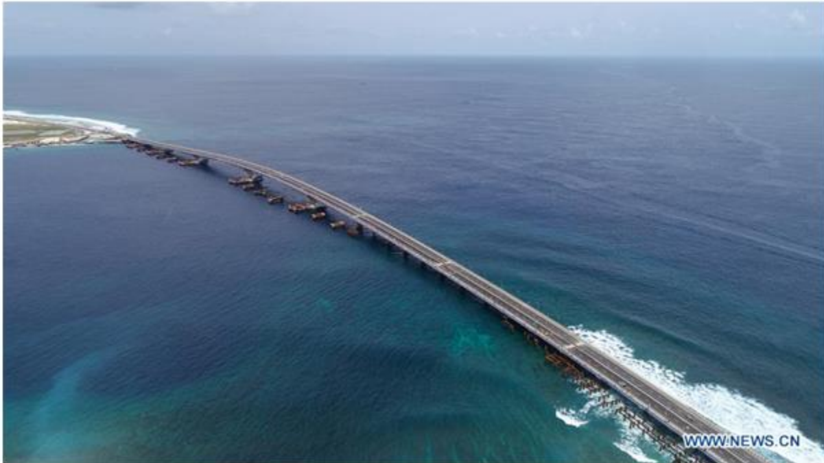
Figure 4: The Bridge of Friendship in Maldives, built by China
